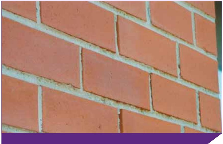
**Figure 12.** Damage to mortar joints by high-pressure cleaning
