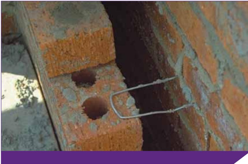
**Figure 11.** Incorrect installation of ties at more than the rated cavity width
