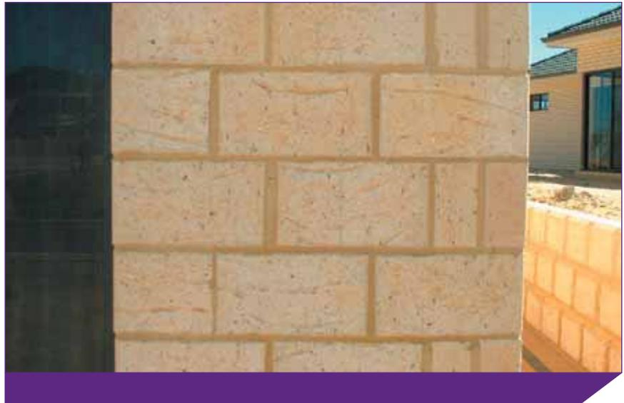
**Figure 14.** Poor control over perpend joint thickness
