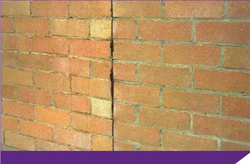
**Figure 9.** Control gap sealant squeezed out by joint closure
