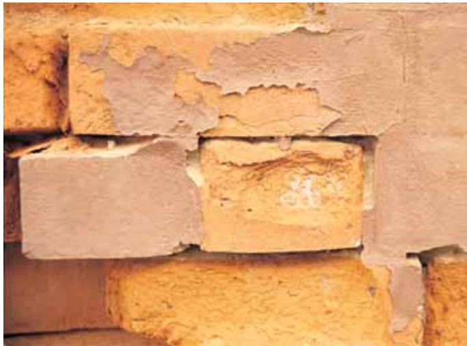
**Figure 13.** Salt attack damage to mortar
