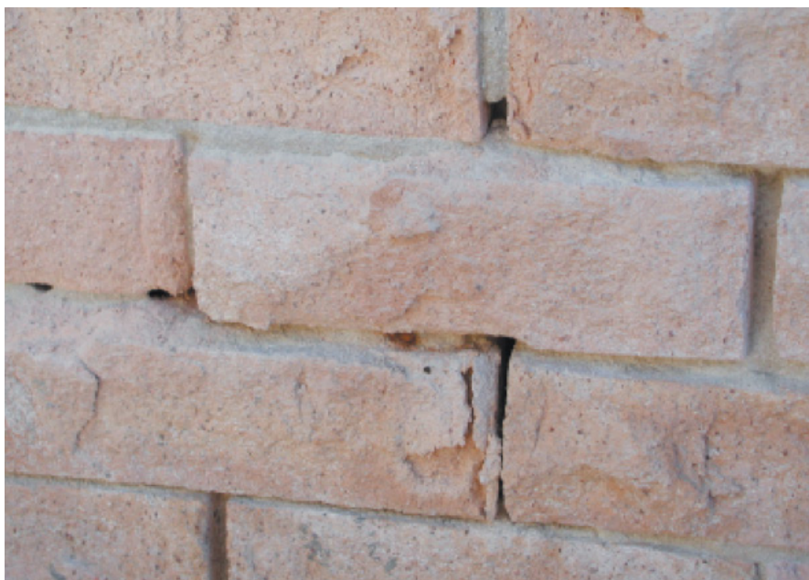
Figure 16. Salt attack damage to clay masonry units
