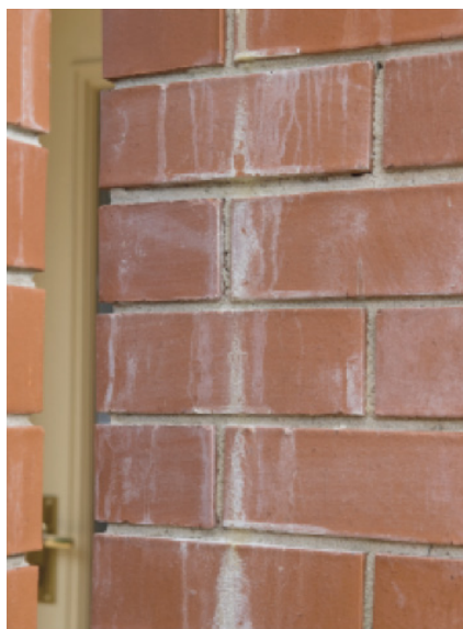
Figure 19. Calcium staining
