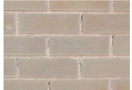
B. Damage to brick face by turbo head
