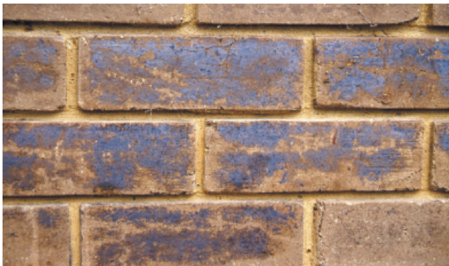
Figure 18. Manganese stains
