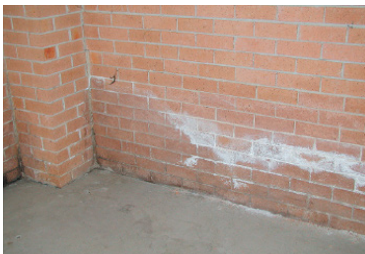
Figure 18. Efflorescence
