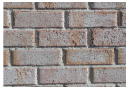
D. Damage to mortar joints
