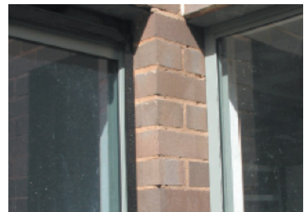
D. Damage to mortar joints
