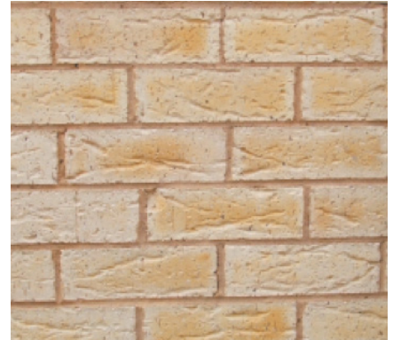
Figure 20. Iron oxide stains
