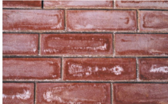
Figure 2. Typical efflorescence from ground salts
