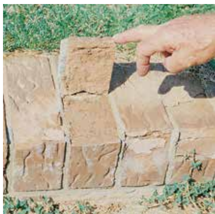
Figure 6. An example of brick delamination due to the effect of freezing and thawing in an Australian alpine area.
