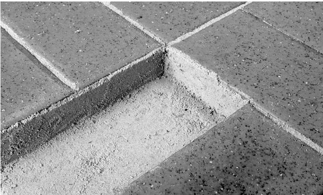
Figure 4 Well-filled sand joint
